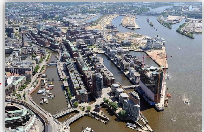
HafenCity in 2017 (© HafenCity Hamburg GmbH)
