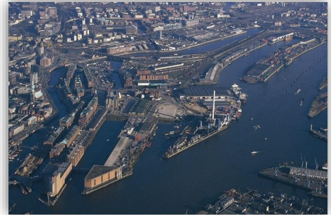
HafenCity in 1997 (© HafenCity Hamburg GmbH)
